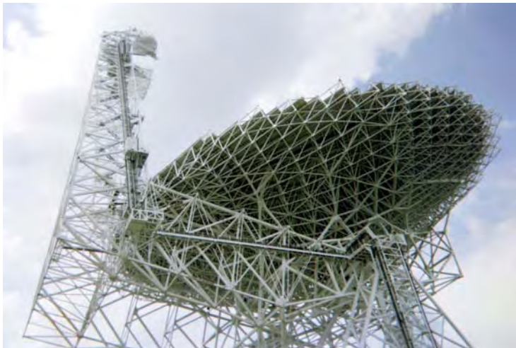
Below: view of the GBT's elevators and cat walk.
